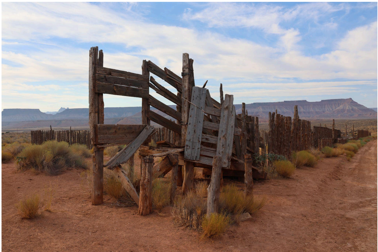
Sheep corral built by CCC men near Zion National Park. Photographed in 2025 by Jeff Nokes
